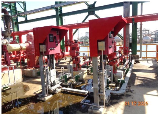
Electric Motor Driven Jockey Pumps
