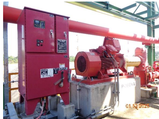
Electrical Driven Fire Water Pump
